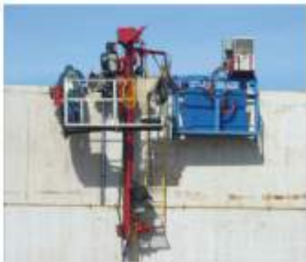
V.U.P Tank Welder
